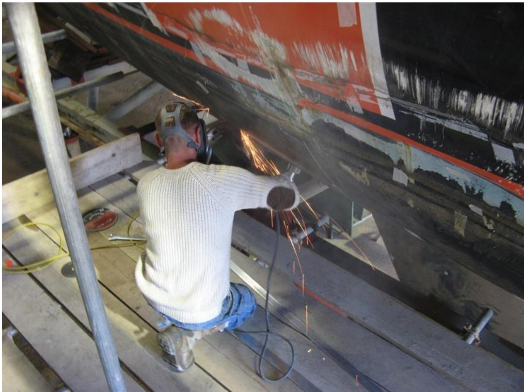
Damaged side plates being cut out
